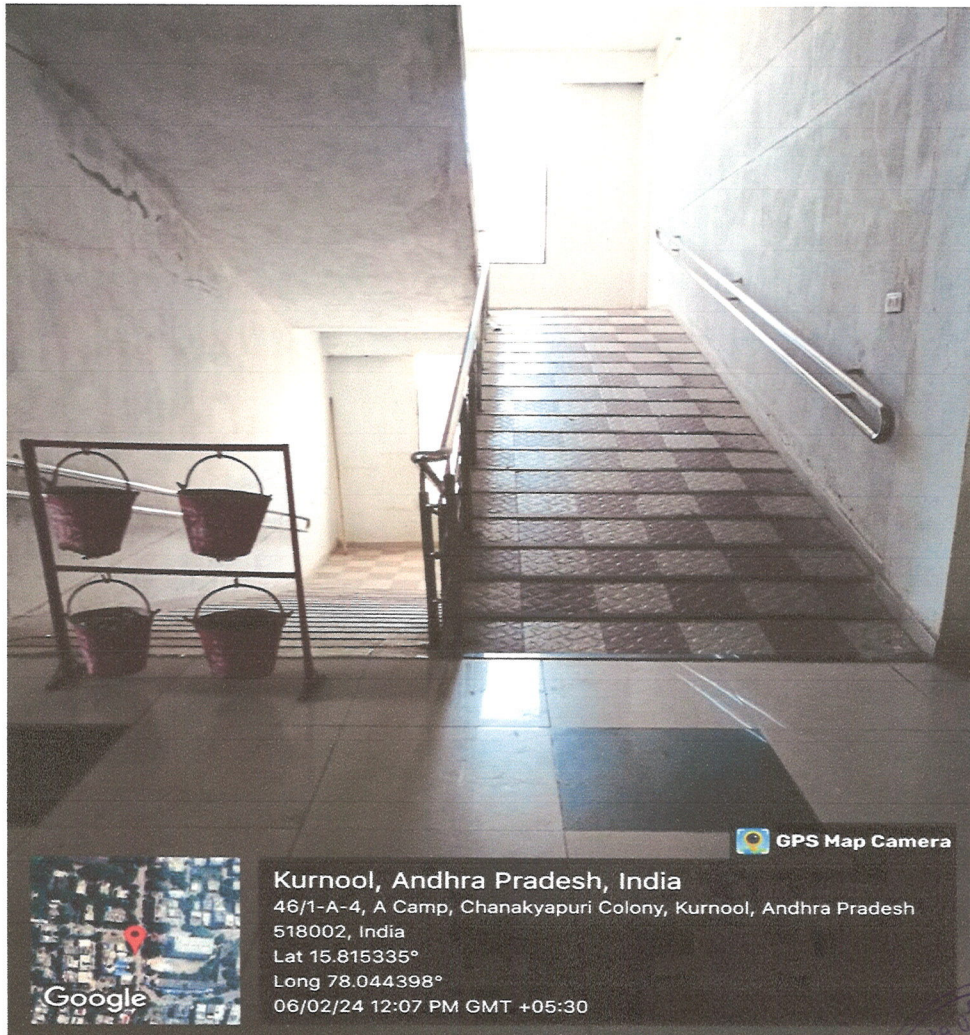
Ramp for disabled students
